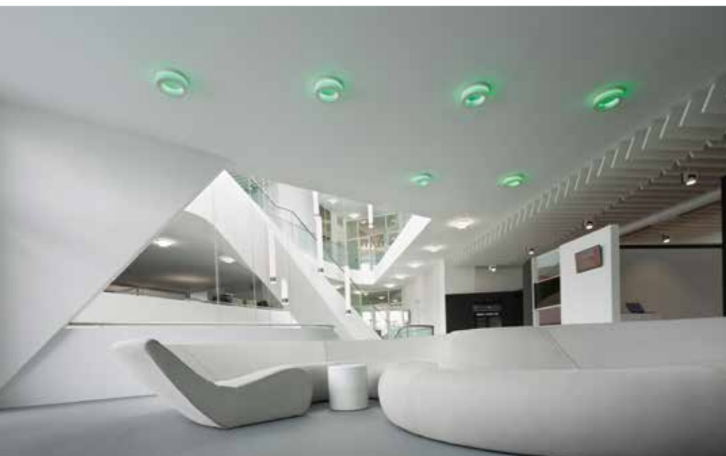
Above: The sides of these pendants emit general light, the downward component illuminates the stairs. Left: Colour-changing fittings in the lounge
