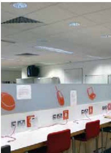
Figure 6.2 Localised lighting over hot desk positions
