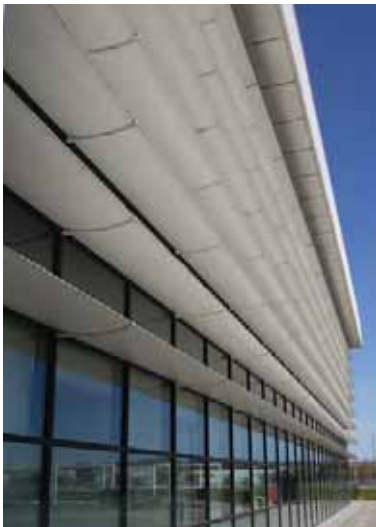
Figure 5.3 Example of horizontal solar shading
