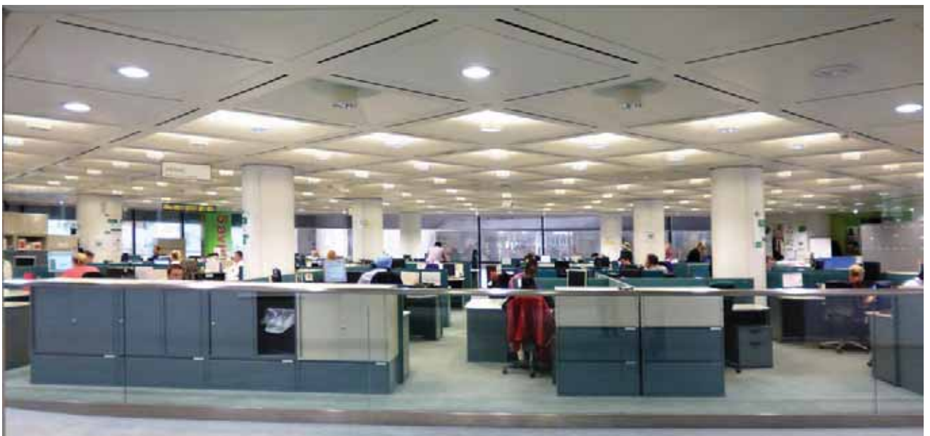
Figure 6.17 Luminaires in coffered ceiling
