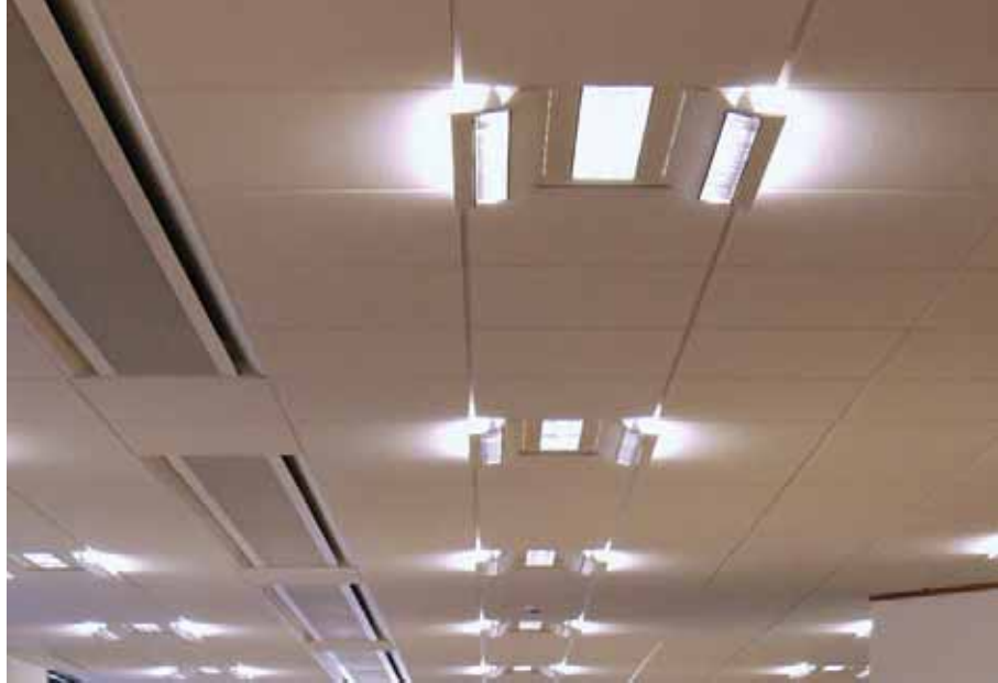
Figure 7.2 Example of lighting and mechanical services coordination
