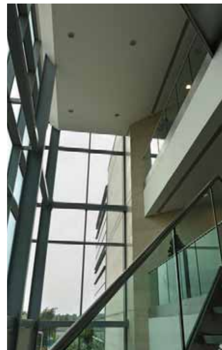
Figure 6.6 Tall space lit with high-pressure discharge lighting
