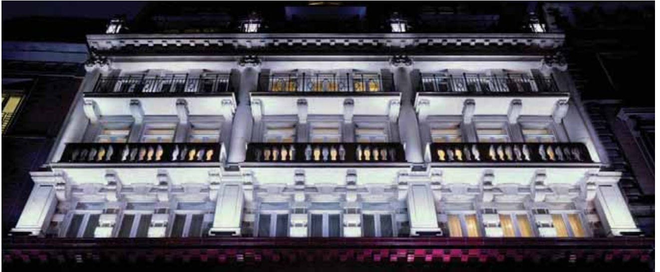
Figure 2.19 Lighting a facade with external recesses (photograph courtesy of it does Lighting Ltd)
