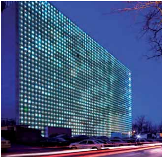
Figure 2.37 The GreenPix facade integrates photovoltaics to achieve a zero-energy balance in operation (photograph courtesy of Arup Lighting)
