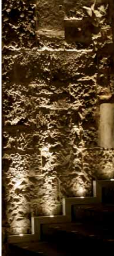
Figure 2.25 Stepped luminaire mounting to uplight a wall (photograph courtesy of dpa lighting consultants)
